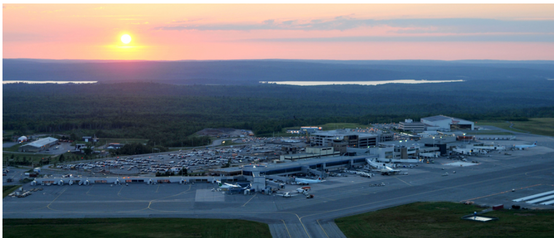
Halifax Stanfield International Airport
